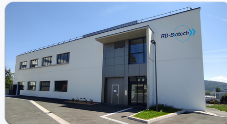
"cGMP PLASMIDS" PRODUCTION FACILITY FULLY OPERATIONAL IN 2023
